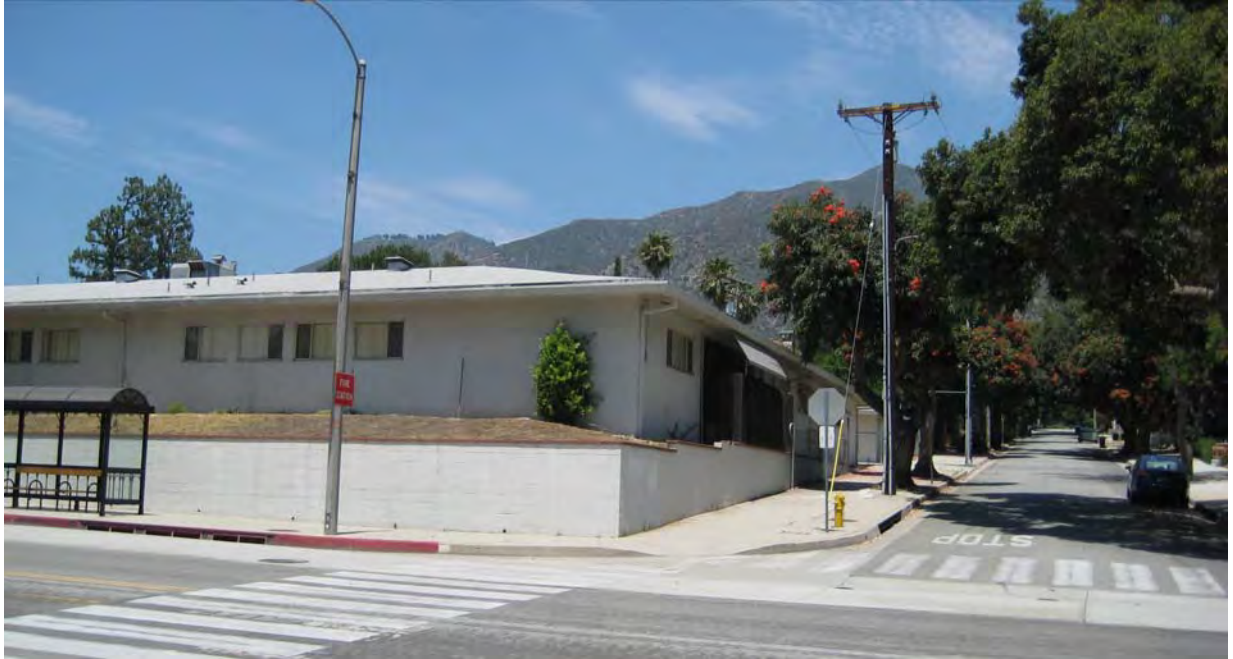
Above: View from southeast corner of Hermosa Ave. and Sierra Madre Blvd looking north
